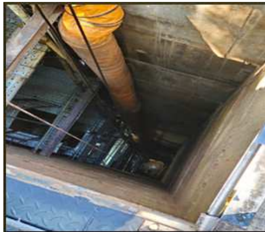
Shaft at Depth
